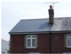
Slate Roof with Chimney Victorian
