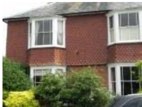
Double Bay Front Sash Windows
