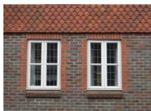
Multi-hue facing bricks, contrasting reveal and soldier course, c.1995
