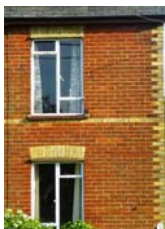
Contrasting quoin and string course c.1880.
