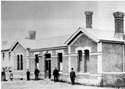
Holmwood Railway Station c.1867. Note the gables, quoins and string course of brickwork.
