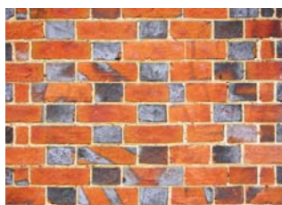
Diaper brickwork c.18 th Century.
