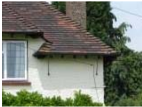
Roof with Plan Tile
