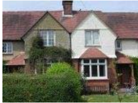
Gable into roof under render/pebbledash
