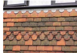
1987, with matching flashing.
