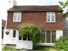
Cottage – render brick under plain roof tile
