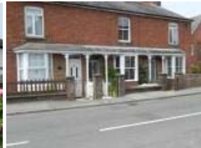
Canopy under brick elevation
