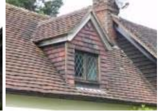
Roof with Dormer
