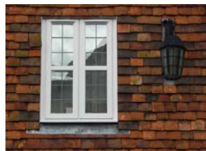
1920's tiles re-hung c.1995
